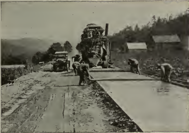
IN CONNECTICUT, ROADS ARE BUILT HALF AT A TIME, AND TRAFFIC IS THEN SAVED A LONGER TRIP OVER AN ALTERNATE ROUTE
